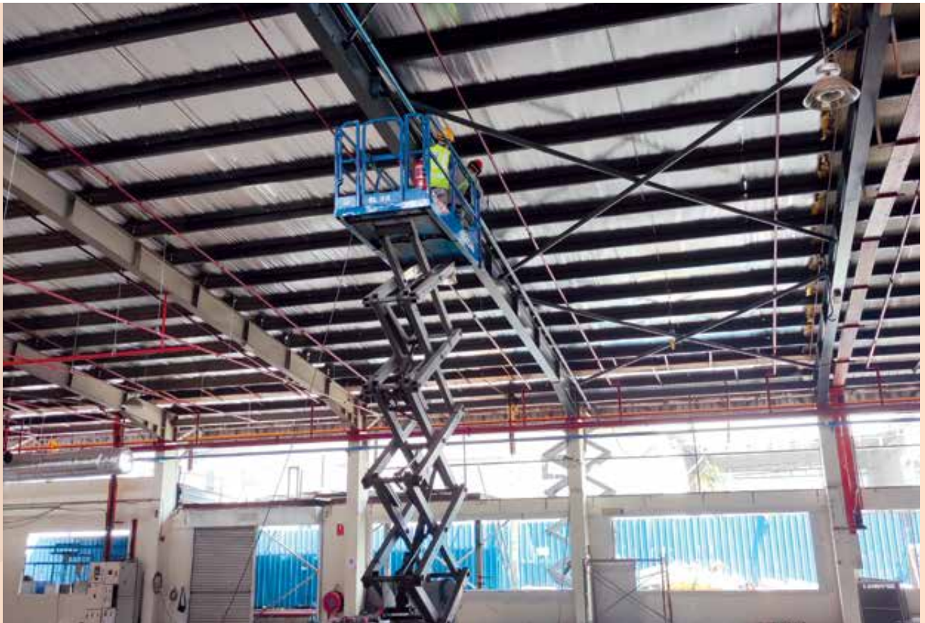
Roofing work progress in August 2022.
